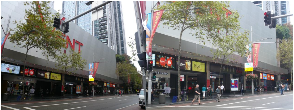
Views of the site from George Street
