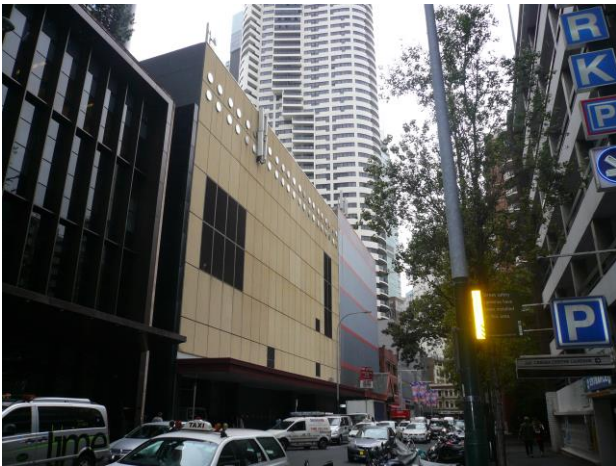
View of the site from Kent Street
