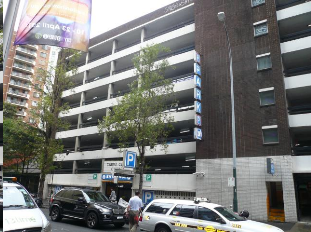
View of Cinema CentreCar Park located on the western side of Kent Street, opposite the site
